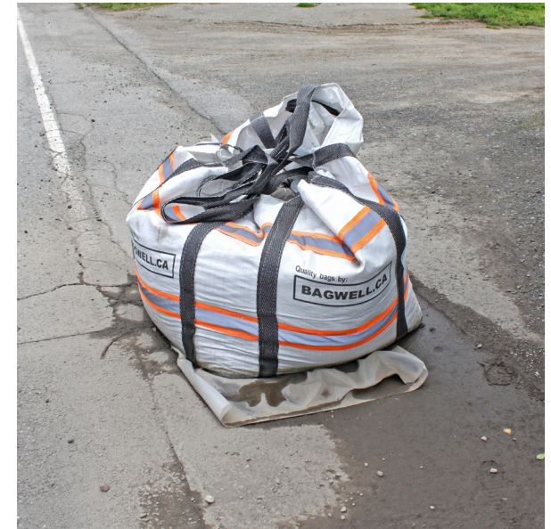
Flood mitigation includes covering drains in low-lying areas
